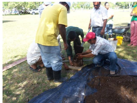
Ensure good compaction of the block
