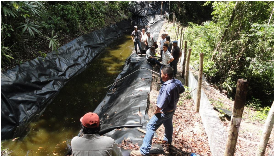
Improved Pond with Geomembrana Plastic & Overflow Gutter – G. Choj's farm
